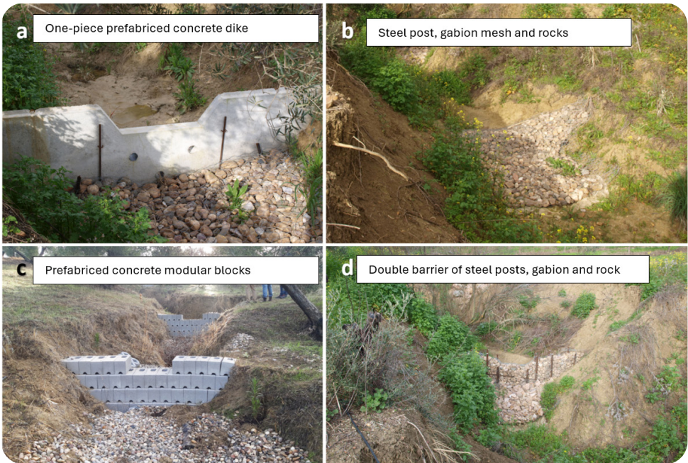
Fig. 1: Control gully dikes with different construction techniques.
